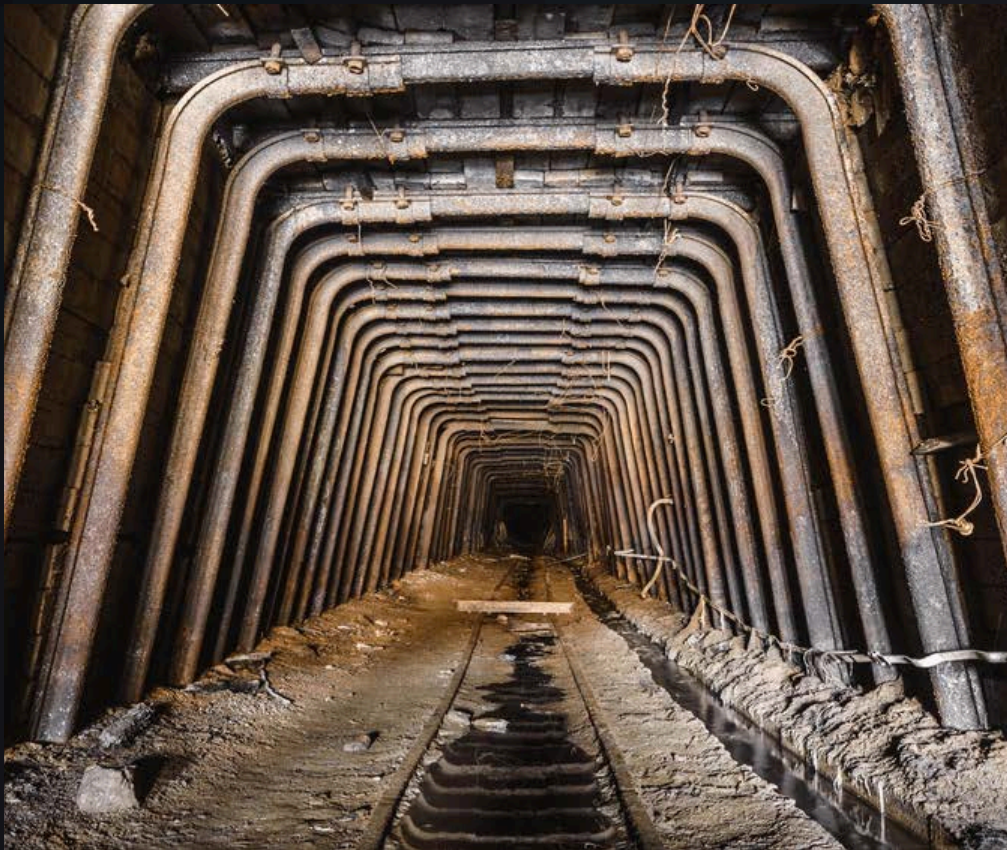
The main portal dating from the 1990s appear to be in fairly good condition.
