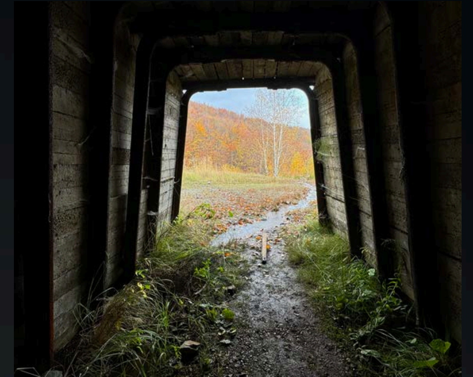
Looking out from the adit
