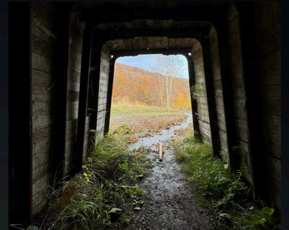
Looking out from the adit
