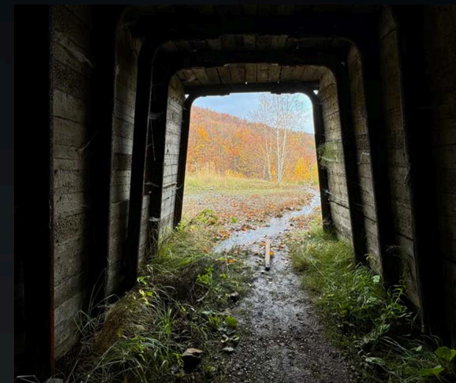
Looking out from the adit
