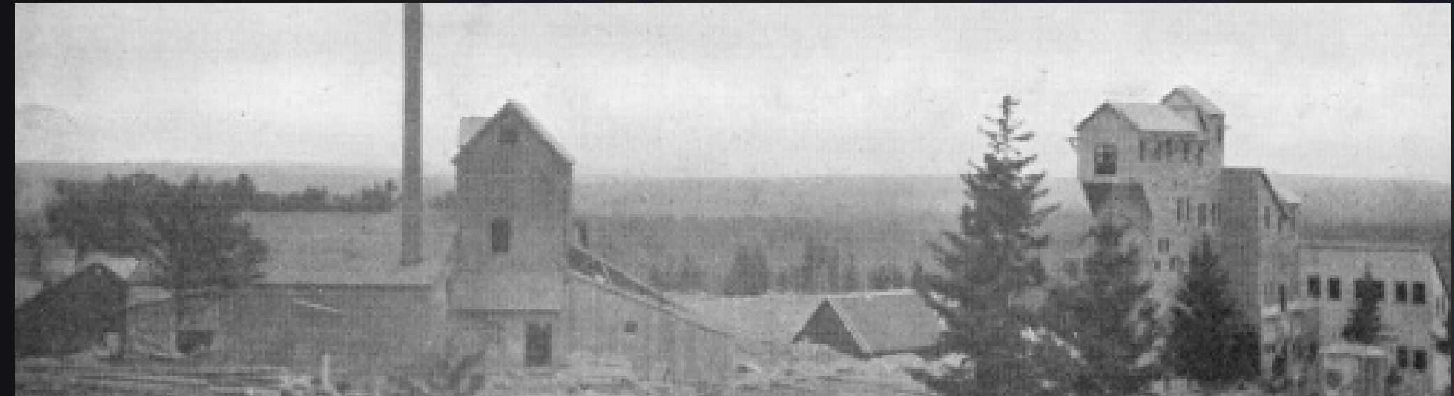
FIGURE 1: Surface workings at West Gore circa 1907 showing the shaft house and the brand new mill building. Source: notyourgrandfathersmining.ca/west-gore
